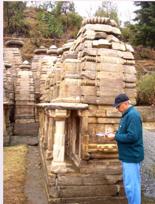
Fig.11a- Northward tilt in miniature Temple
