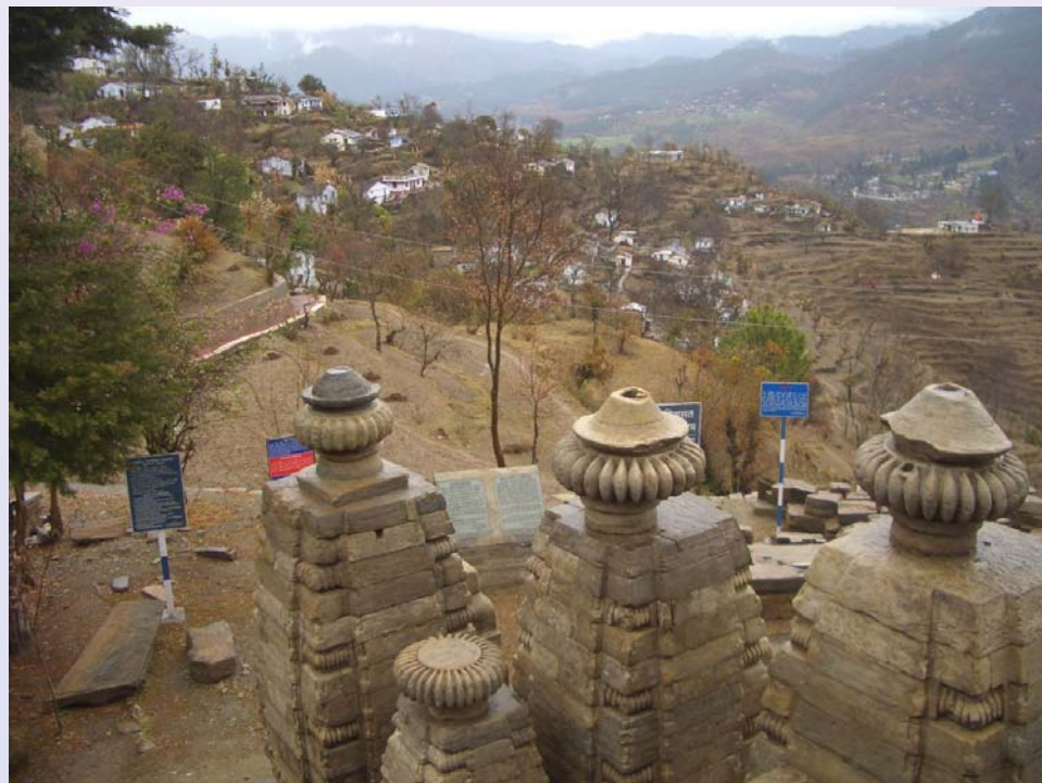
Fig.11b - Displaced shikhars of the miniature temples
