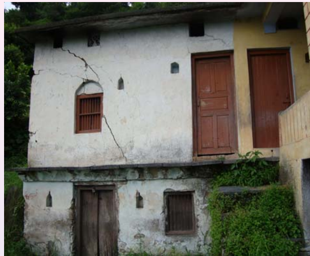
Fig.4-Road subsidence and damaged houses
