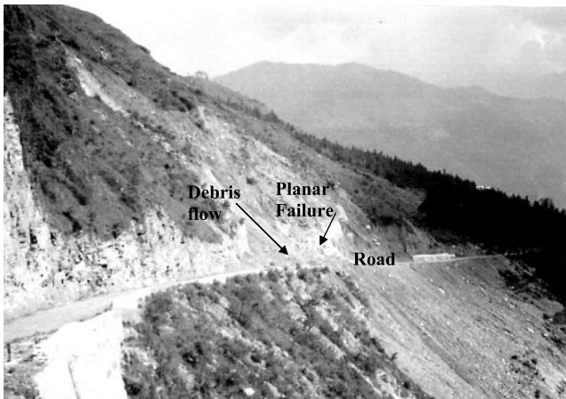
Fig. 5. View of landslide 1 showing multiple failure modes.
