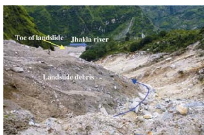
Figure 4. Debris accumulation on downhill slope below road level.
