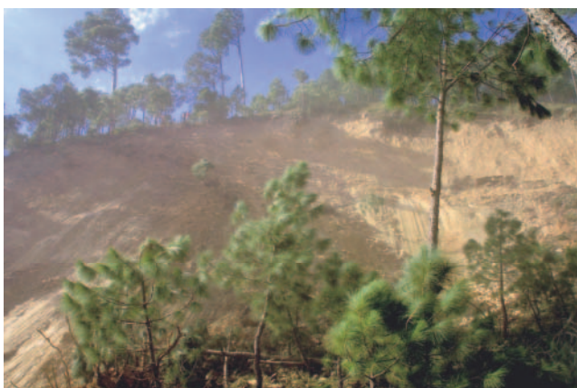
Fig. 2. Main escarpment of the landslide.
