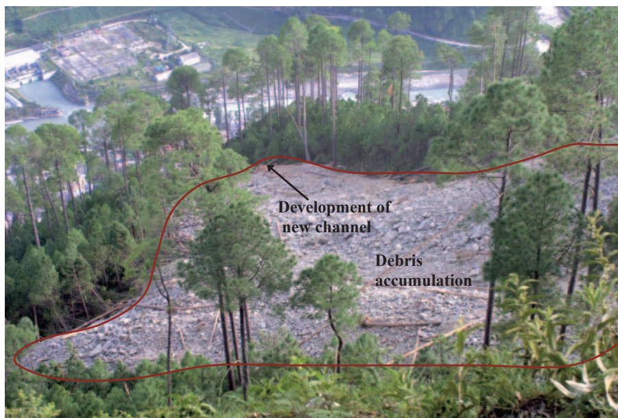
Fig. 7. Development of new channel for debris slide and rock fall.
