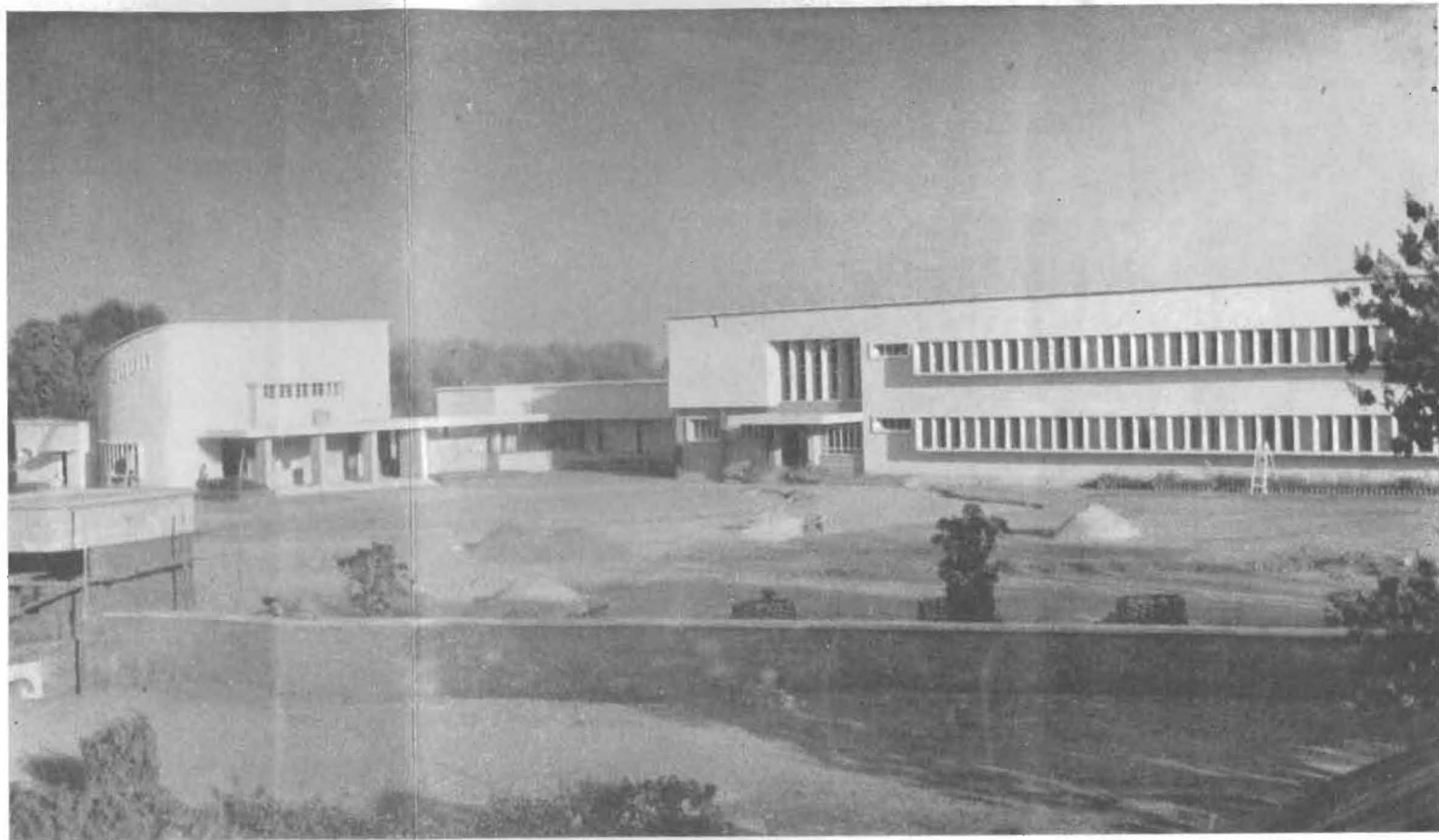
Central Building Research Institute, Roorkee
