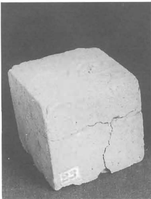
Fig. 11. Concrete cube having uncoated MS rebars (80 cycles).
