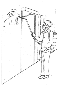
Fig. 3 Spraying of Termiticide Emulsion
