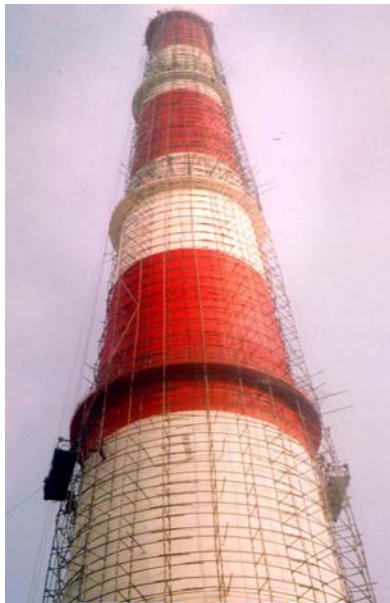
Figure 9 A chimney after repair and coating
