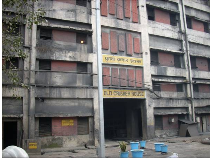
Figure 2 A crusher house building
