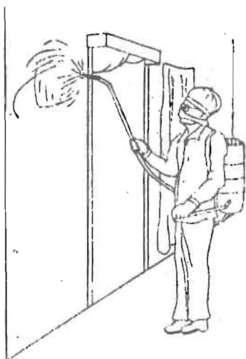
Fig. 3 Spraying of Termiticide Emulsion
