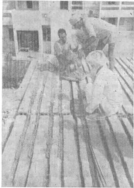
Fig. 4. Placing Concrete in the Clay Unit Slab Assembly 1446 P.P.
