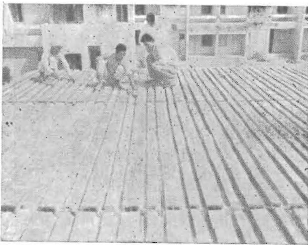
Fig. 3. Clay Units Laid Between Joists 1448. P.P.
