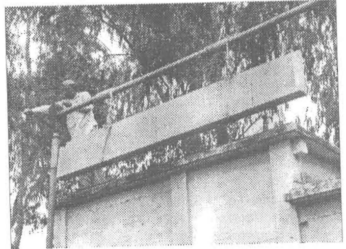
Plate 5 — Innovative winch-Hoist for Erection of L-Panels
