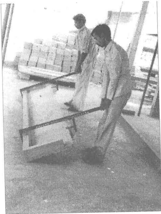
Plate 4 — Safe Lifting of L-Panels from Platform
