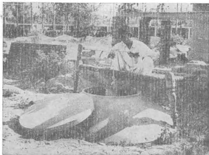
Fig. 8 Semi Underground Cement Bin Capacity 1 Tonne
