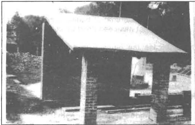
Fig. 2 : Finished Thatch Roof
