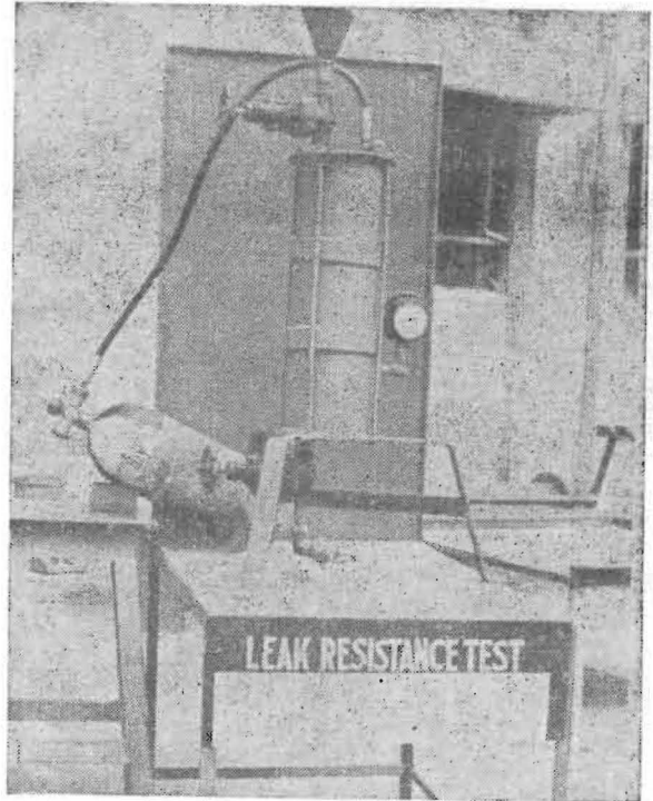
Fig. 3 Leak Resistance Test Apparatus
