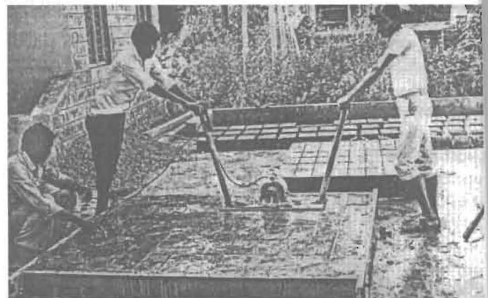
Fig. 9 Casting of Blocks with multi-pockets Gand Mould
