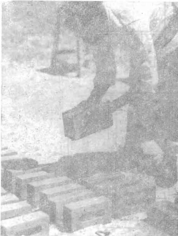
FIG. 4. BRICK BEING PLACED ON EDGE FOR DRYING.
