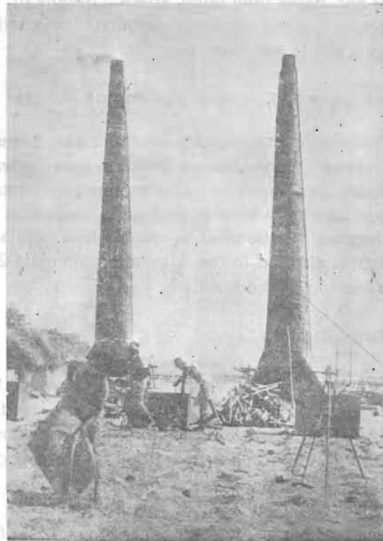
Photo—Feeding of Rice Husk in Commercial Bull's Trench Kiln.
