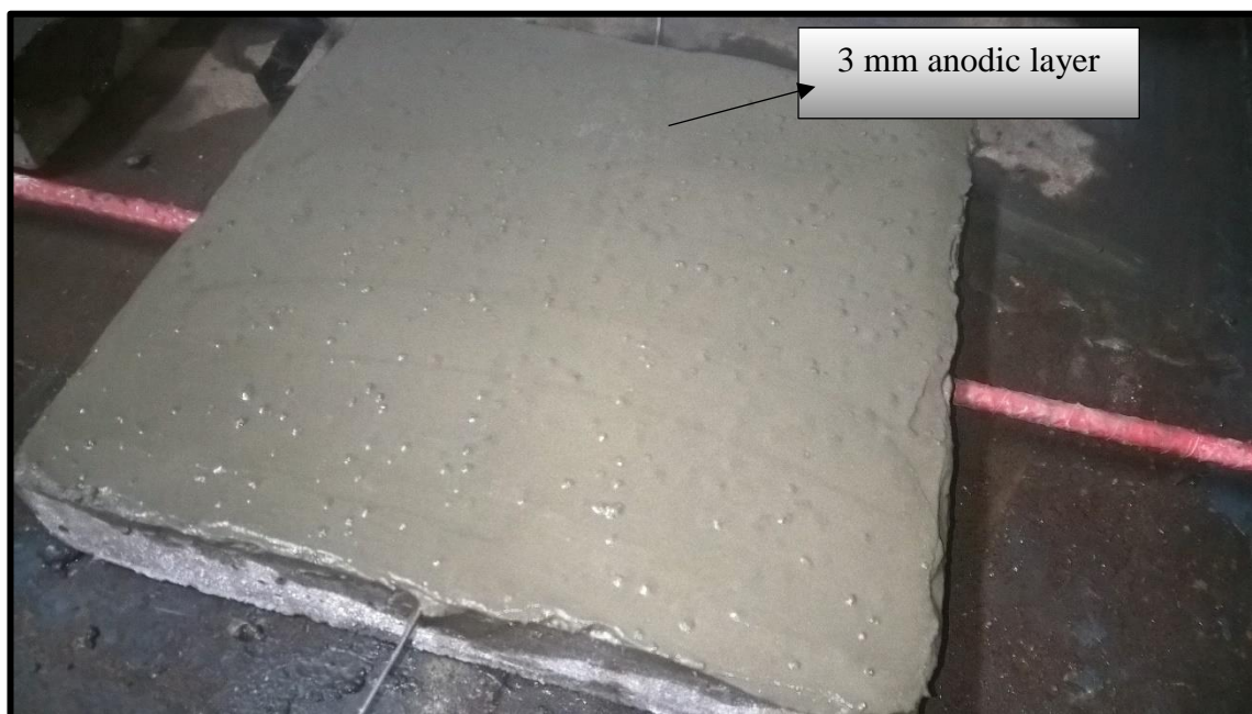
Figure 3.15 Application of anode layer on concrete slabs
