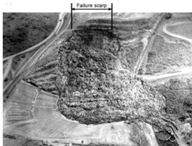
Fig. 1.2 Failure of bulbul landfill in Durban, South Africa (Blight, 2008)
