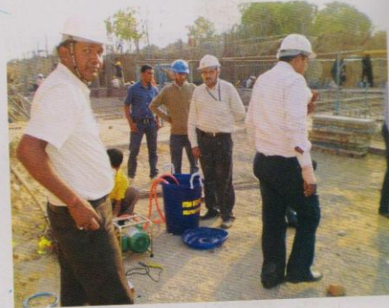
Photo 23: Installation work of Item Secure Technology at construction site in Ahmedabad
