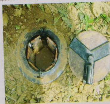
Photo 11: Internal view of an IGBS with wooden interceptors
