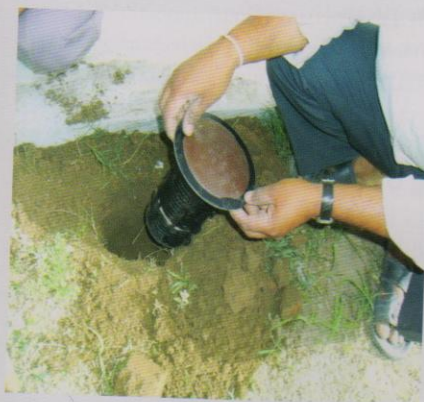
Photo 13: Complete IGBS before installation
