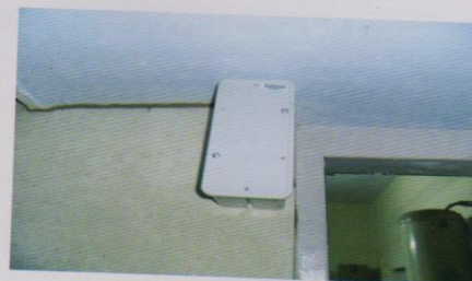
Photo 14: AGBS after installation on wall
