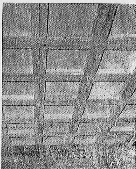
Fig. 5 Ceiling of waffle unit roof
