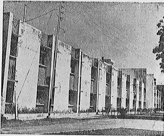
Fig. 2. Exterior algae growth on parapets.
