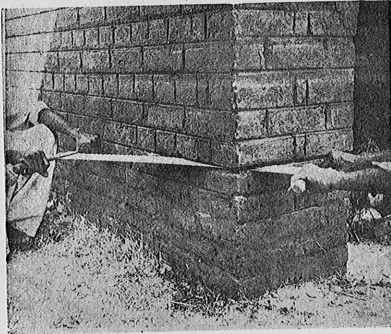
Fig. 2. Starting the cut at a corner
