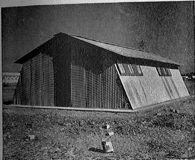
Fig. 1 Completed prefabricated hut
