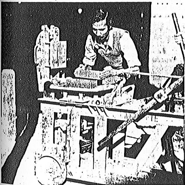
Moulding stabilized soil bricks in a Landcrete machine
