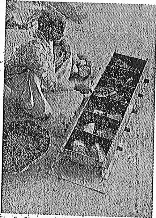
Fig. 5. Casting of Stone Masonry Blocks (Stone Spalls with Concrete at bottom)
