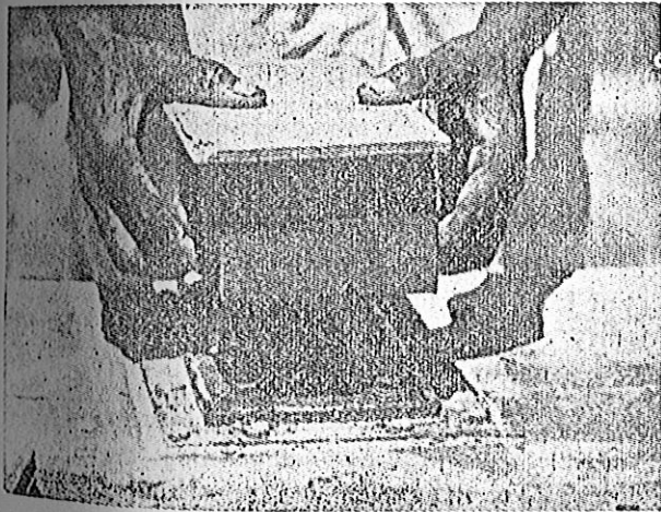
Fig. 3 Removing Brick from Mould
