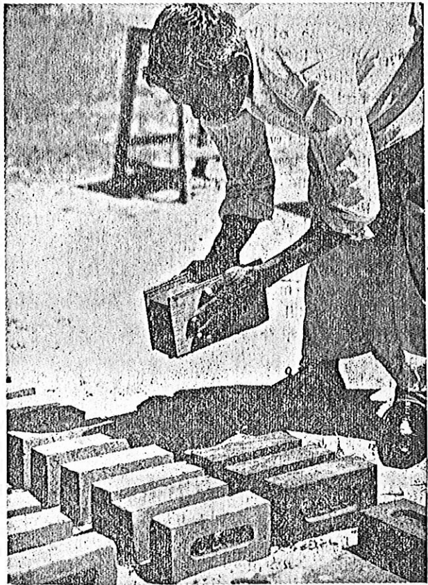
Fig. 4 Placing Brick on Edge for Drying
