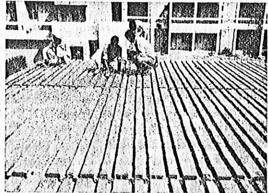
Fig. 10 Construction of roof (joist and Infill type) using structural clay products
