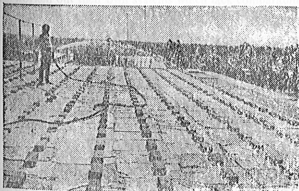
Fig 21 Roof spray method of cooling of buildings
