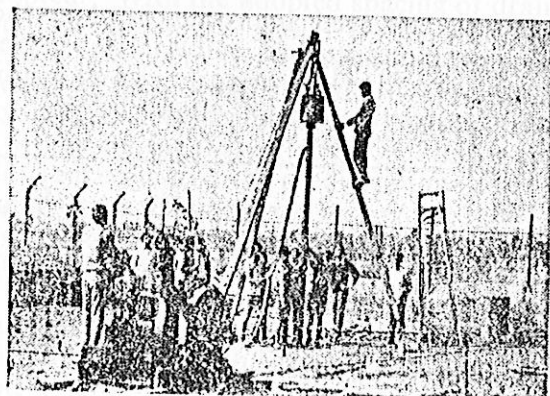
FIGURE 4 Driving operation for installation of rope drains.
