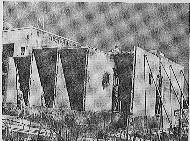
Fig 5 Cross-wall panels erected
