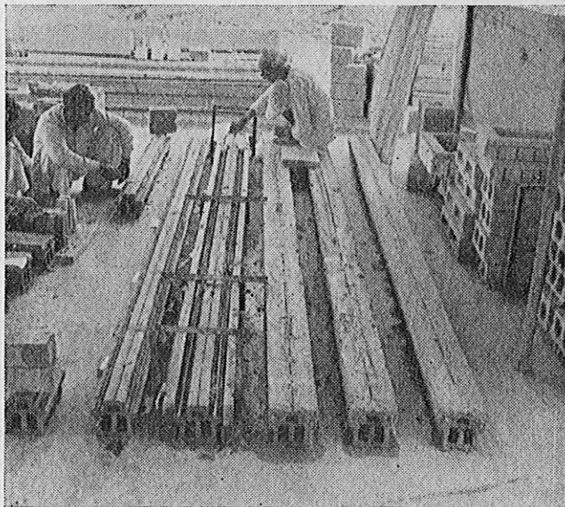
Fig 2 Different stages of prefabrication of joists
